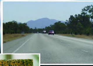
Good roads are fundamental for sustainable development
