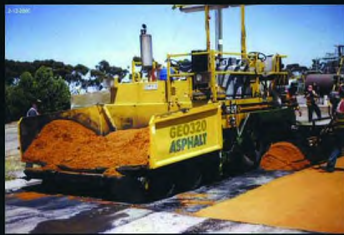
EcoPave GEO 320 being applied
